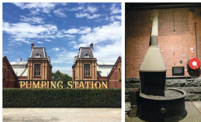
Spotswood Sewage Pumping Station at ScienceWorks
