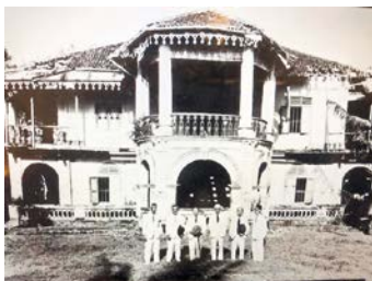
The dilapidated villa with the six SCCCI council members in front
